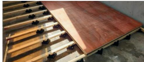
Installing Acoustic underlay for Better Performance (Cradle + Batten + Plywood + Underlay + Plywood)
